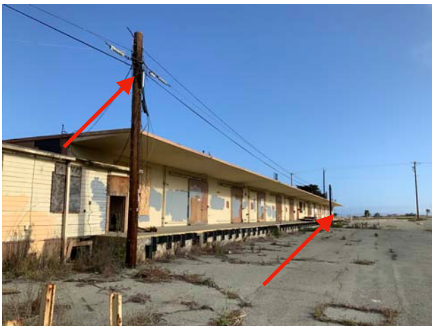
T2064/2065 - Utility Poles & Wires
