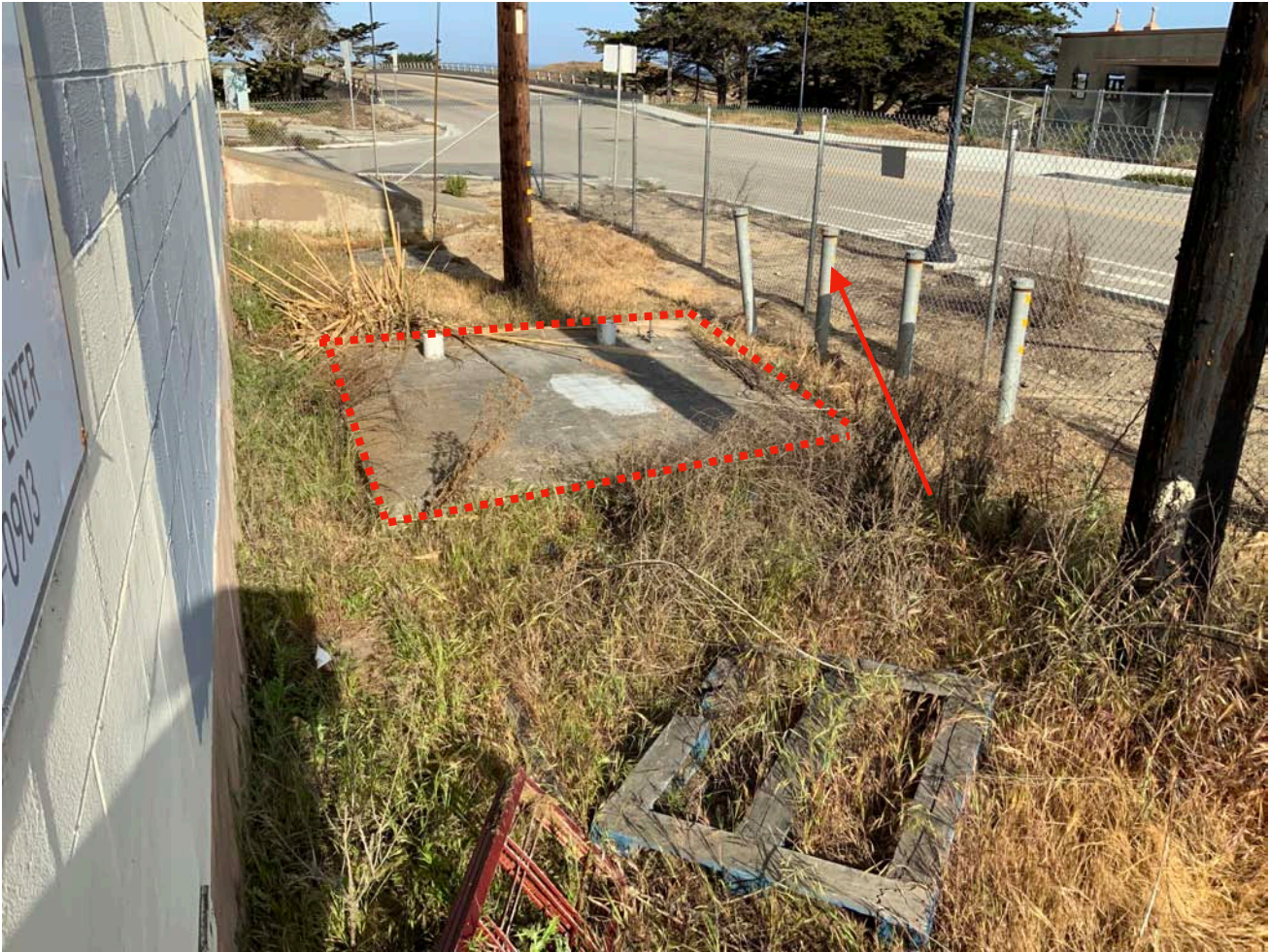
T2065 - Transformer Pad & Bollards
