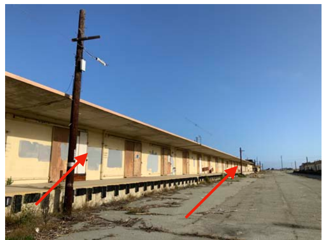
T2063 - Utility Poles & Wires
