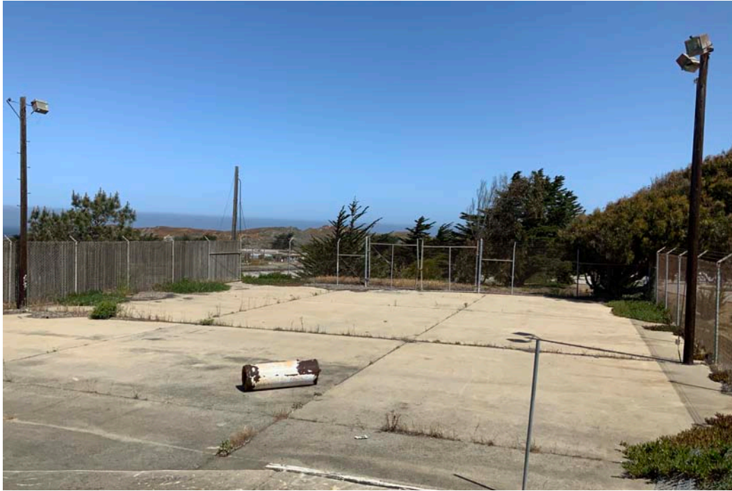
T2071 - Slab, Fence, and Light Poles
