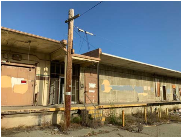
T2060 - Utility Pole & Wires
