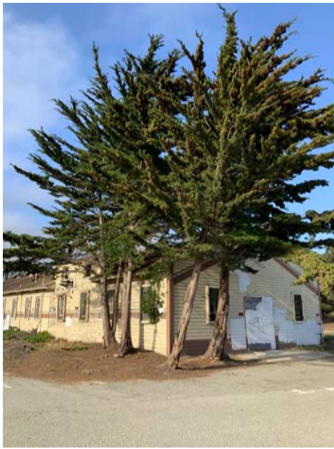
T2058 - Trees in Demolition Limits
