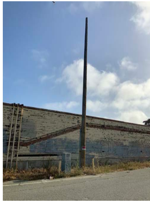
T2060 - Utility Pole, Box and Bollards in Demolition Limits
