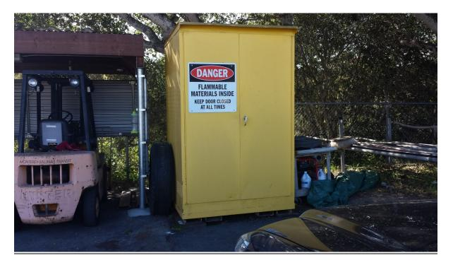
Photo 20 – Liquid Flammable Materials Storage
