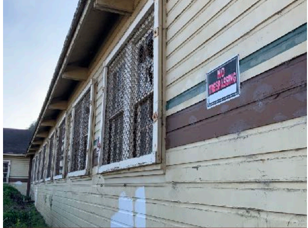
Defective Lead-Based Paint On Exterior Siding & Window Components
