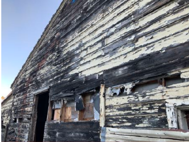
Defective Lead-Based Paint On Exterior Painted Wood Components
