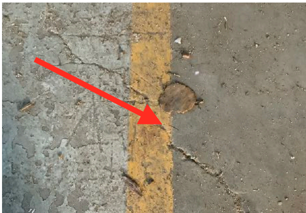
Warehouse Area - Yellow Striping With Lead-Based Paint On Concrete
