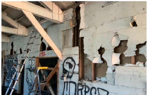
Warehouse Area - Defective Lead-Based Paint On Wood & Drywall, Walls & Ceilings
