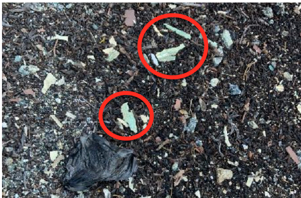
Paint Chips With Lead-Based Paint Present In The Soil Near The Building
