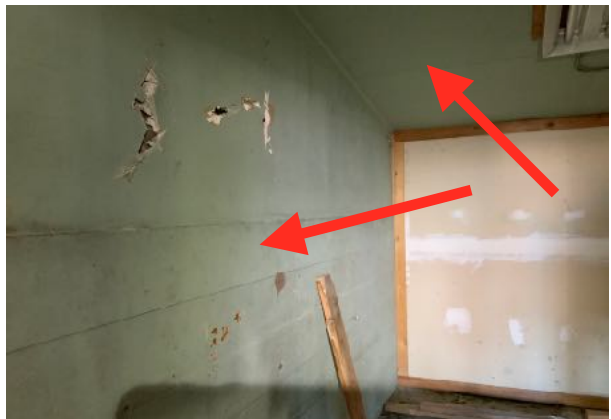
Storeroom #1 - Lead-Based Paint On Walls & Ceiling
