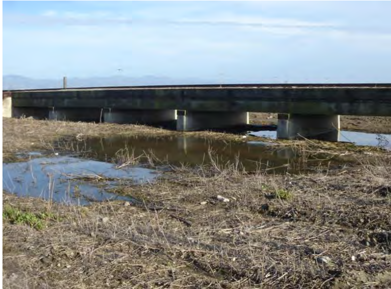
Figure A-25. Floodplain Equalizer Timber Trestle Bridge at MP 113.04
