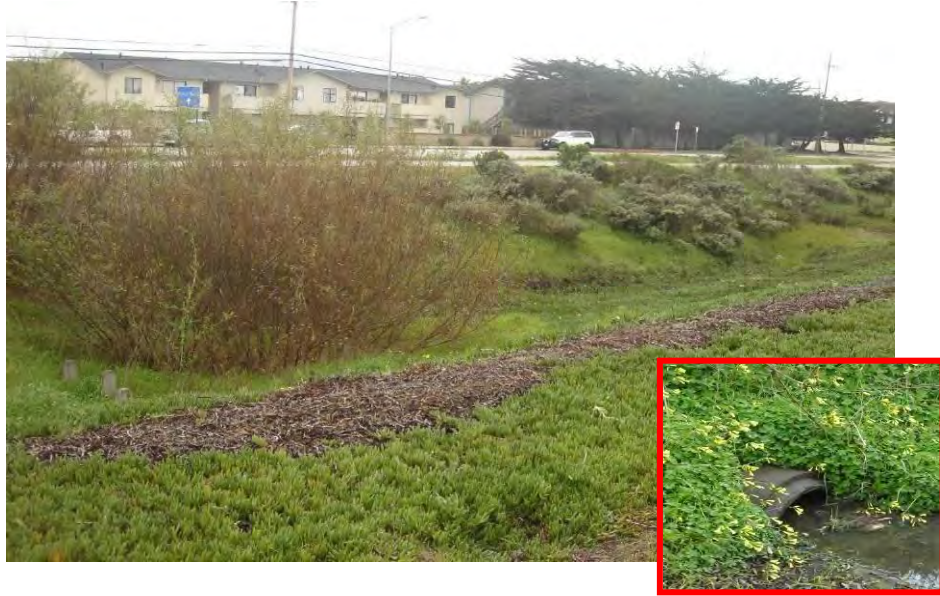
Figure A-39. Swale at the Southeast of Marina Green and Rail with a Culvert
