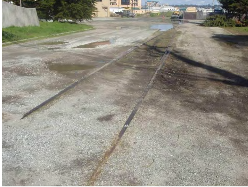
Figure A-56. Ponding North of Contra Costa Street Crossing
